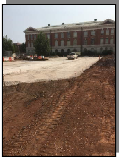
PICTURED ABOVE: EXTERIOR SE SITE GRADING
