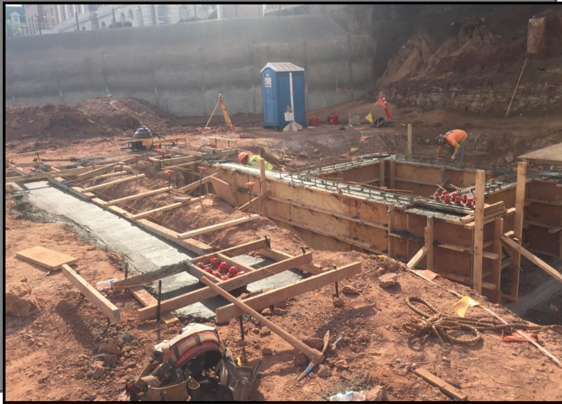
PICTURED ABOVE: FORMED ELEVATOR PIT
