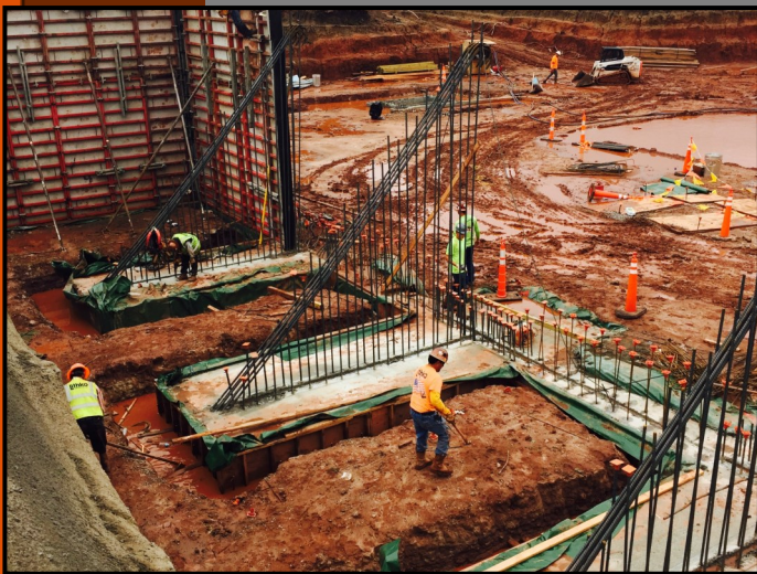
PICTURED: LITHKO FORMING/ POURING FOUNDATION, BASEMENT WALLS, & COUNTERFORT WALLS
