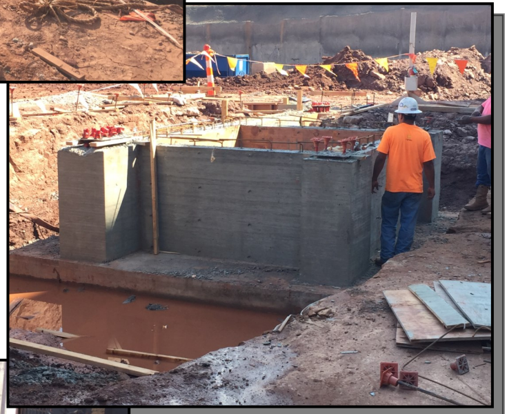
PICTURED ABOVE: FORMED ELEVATOR PIT
