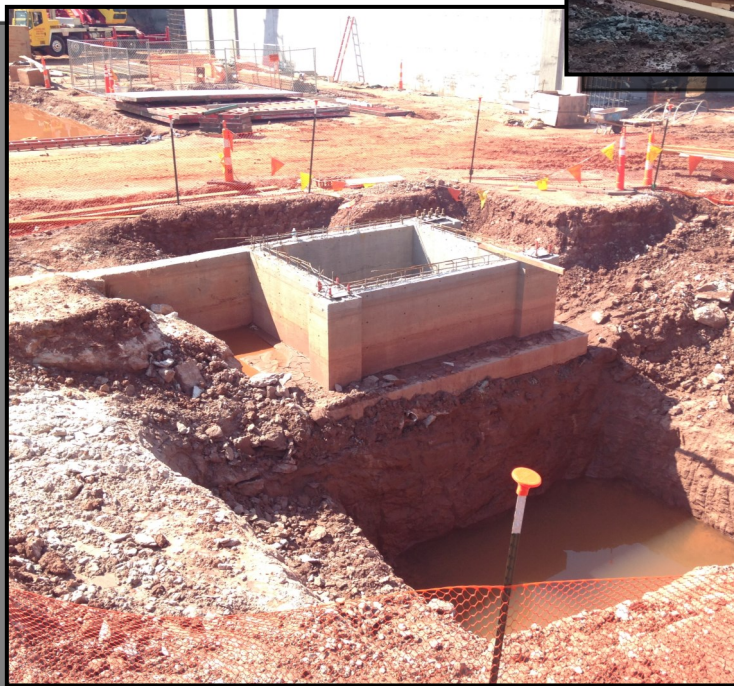
PICTURED LEFT: NORTH ELEVATOR PIT/SUMP BASIN
