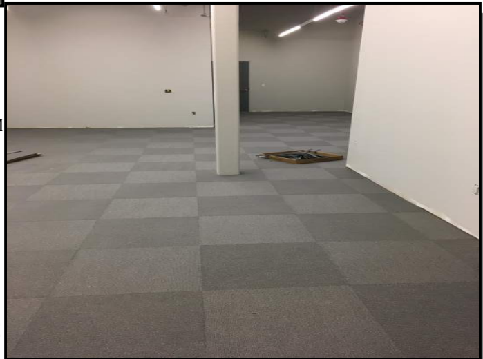
PICTURED BELOW: 4TH FLOOR SOUTH STAIRWELL TILE INSTALLED
