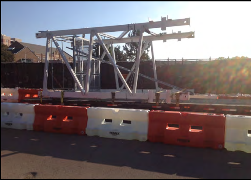
PICTURED LEFT: ARRIVAL OF TOWER CRANE BASE
