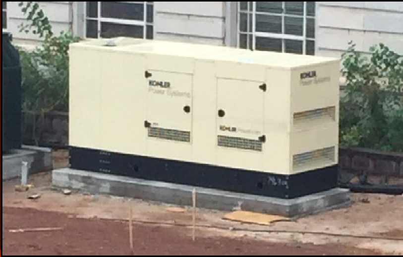
PICTURED ABOVE & BELOW: GENERATOR INSTALLATION
