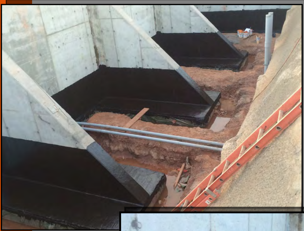
PICTURED: BFF WATERPROOFING BASEMENT WALLS ALONG HESTER ST.
