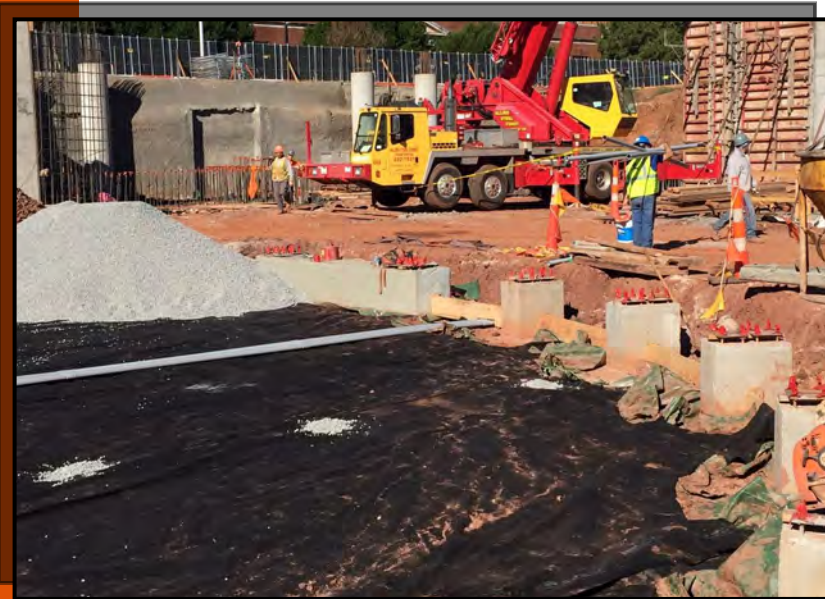
PICTURED LEFT: FORMING 2'-3" DEPRESSED SLAB
