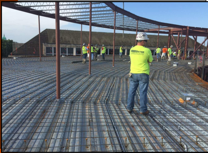
PICTURED: BEFORE AND AFTER PICTURES OF THE LIGHTWEIGHT CONCRETE PLACEMENT ON THE 4TH FLOOR SOUTH HALF SOMD
