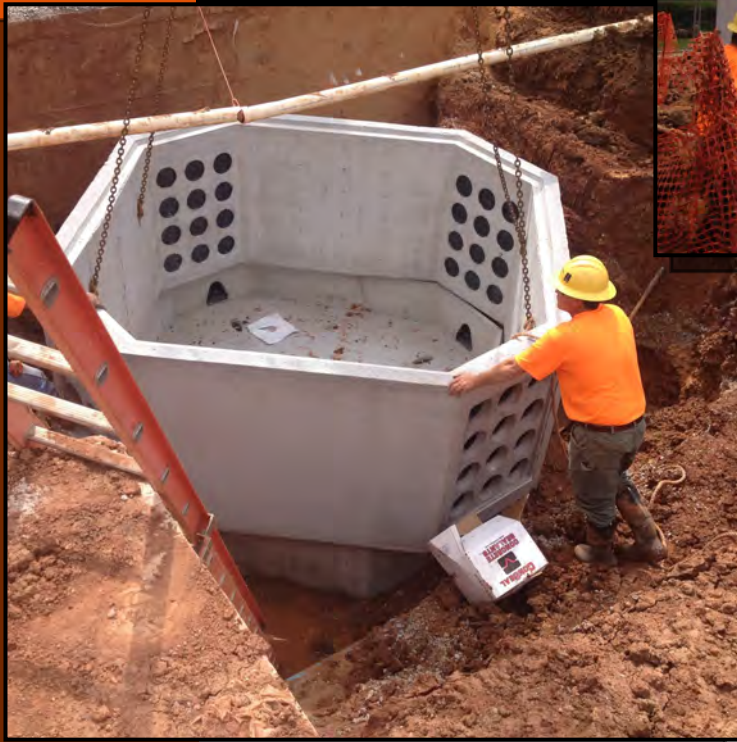
Pictured: The installation of Morrill Street electrical vault
