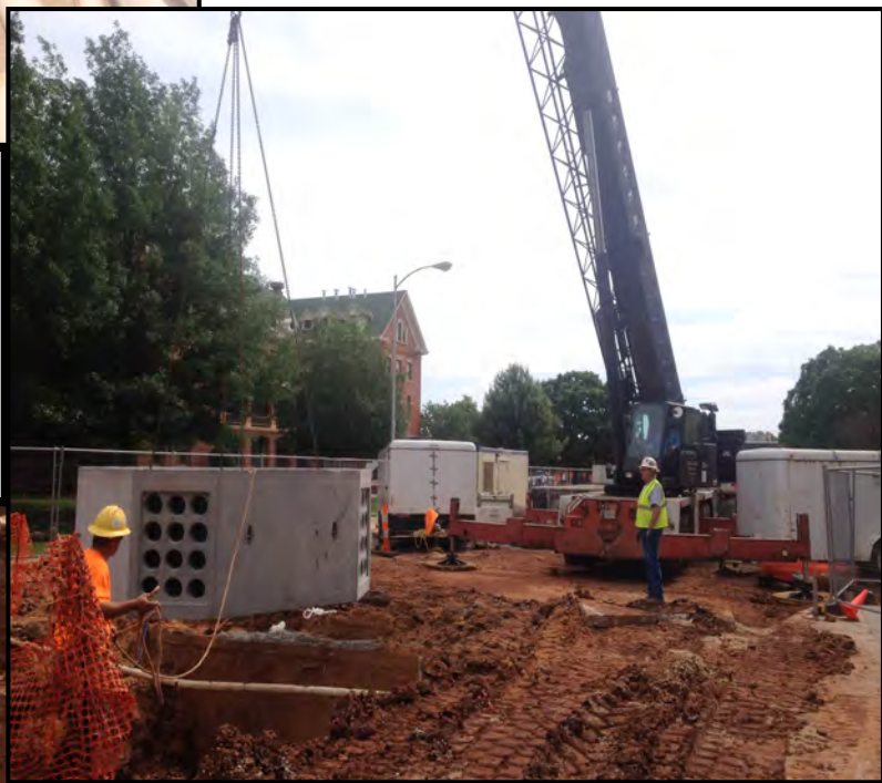
Pictured: The installation of Morrill Street electrical vault
