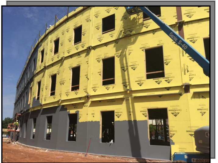
PICTURED: NEWLY INSTALLED EX- TERIOR FRAMING, SHEATHING, AND WEATHER BARRIER ON THE SOUTH & EAST SIDES OF THE NEW BUILDING
