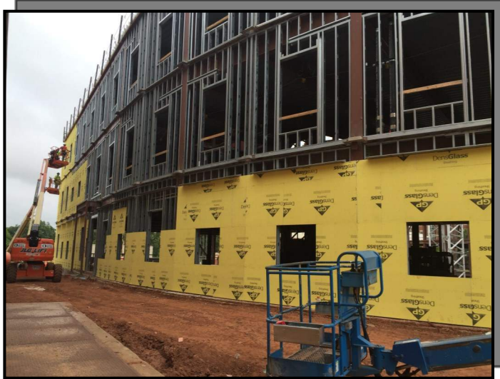
PICTURED: NEWLY INSTALLED EX- TERIOR FRAMING, SHEATHING, AND WEATHER BARRIER ON THE SOUTH & EAST SIDES OF THE NEW BUILDING
