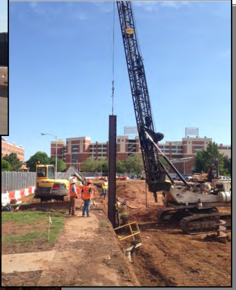
PICTURED: PLACEMENT OF PILES FOR RETENTION SYSTEM
