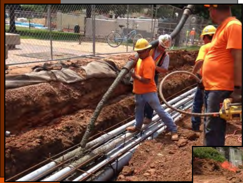
PICTURED: ELECTRICAL DUCT BANK ON THE EAST SIDE OF MORRILL
