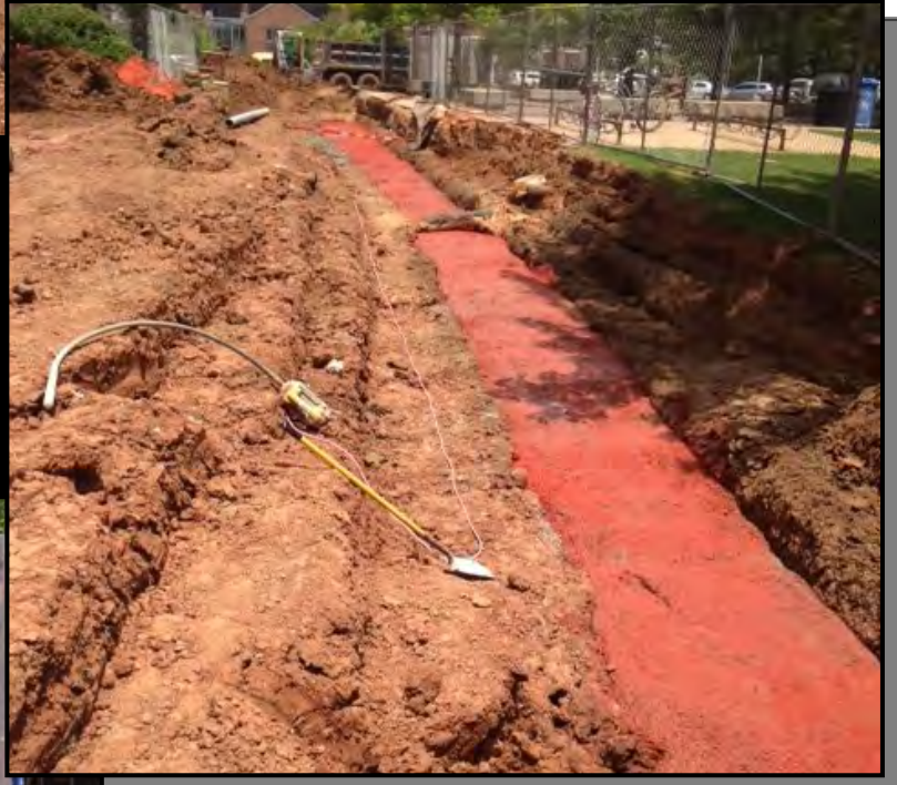
PICTURED: ELECTRICAL DUCT BANK ON THE EAST SIDE OF MORRILL
