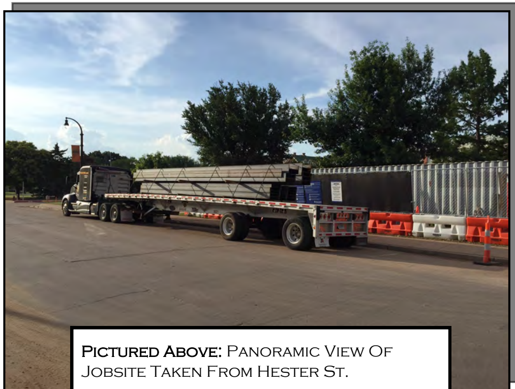
PICTURED BELOW: ARRIVAL OF STEEL FOR RETENTION SYSTEM
