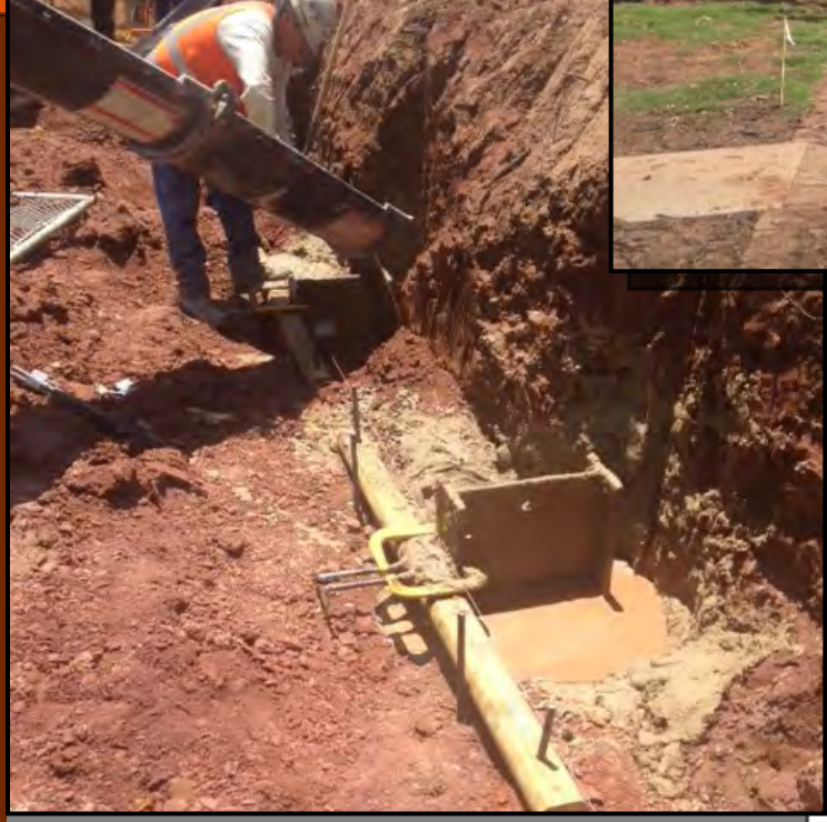
PICTURED: PLACEMENT OF PILES FOR RETENTION SYSTEM
