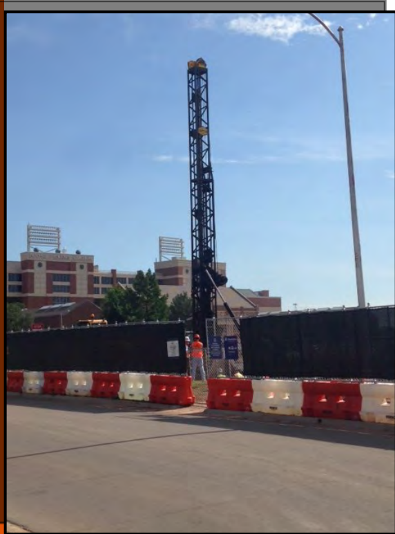
PICTURED: PLACEMENT OF PILES FOR RETENTION SYSTEM
