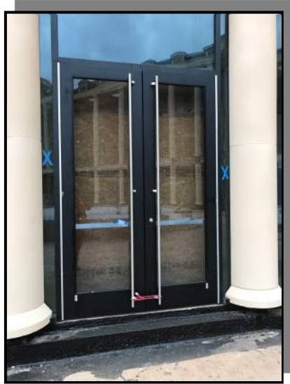
PICTURED ABOVE: EXTERIOR LOGGIA DOORS
