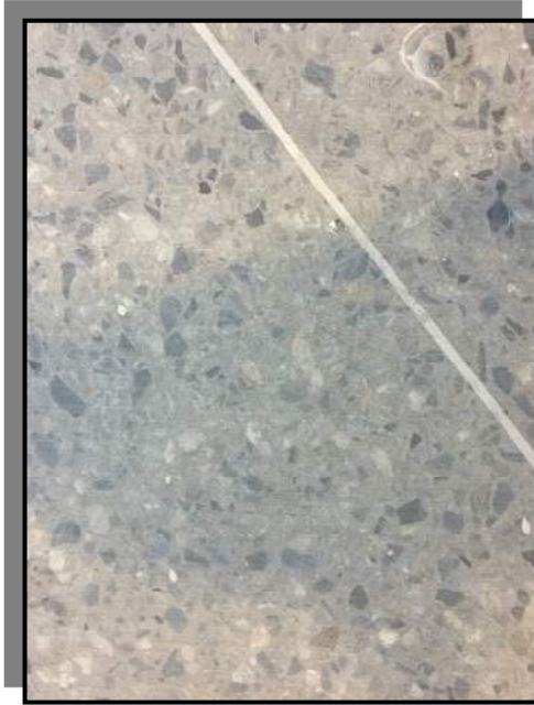
PICTURED ABOVE: 4TH FLOOR TERRAZZO GRINDING
