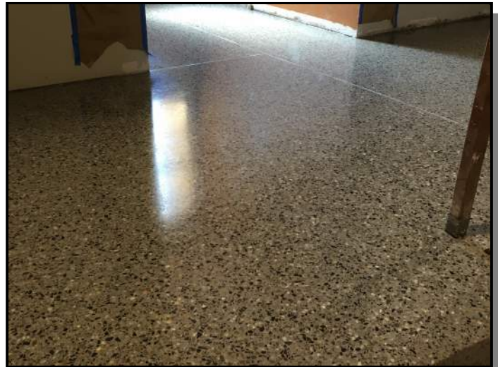
PICTURED ABOVE: 4TH FLOOR TERRAZZO GRINDING
