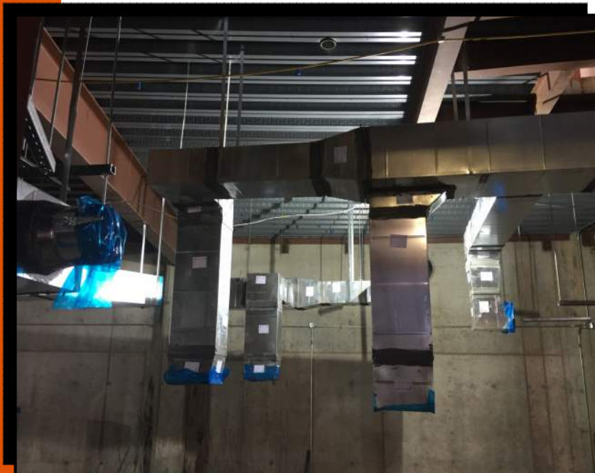
PICTURED: DUCTWORK INSTALLATION IN THE BASEMENT
