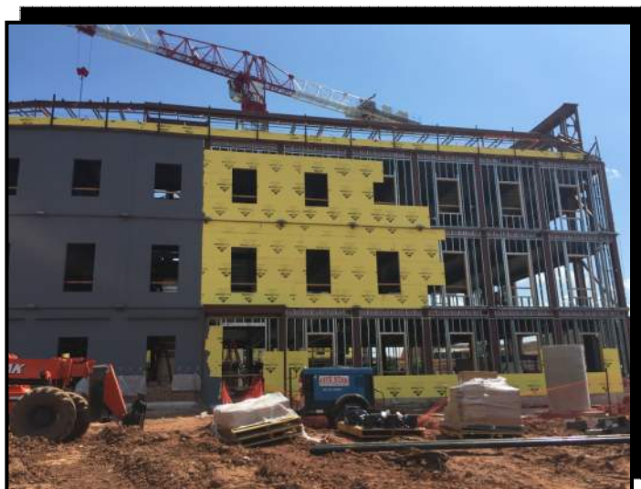
PICTURED ABOVE & RIGHT: WEATHER BARRIER, SHEATHING, AND FRAMING ALONG THE NORTH AND EAST EXTERIOR WALLS
