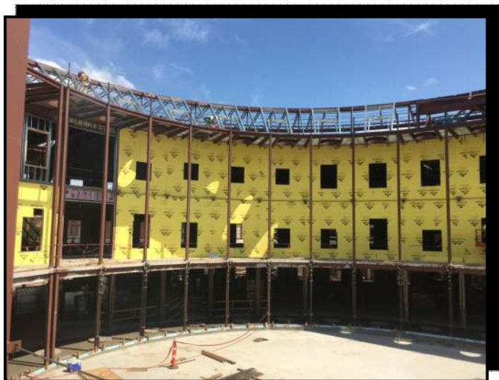
PICTURED BELOW: SHEATHING AND FRAMING ON THE SOUTH SIDE INTERIOR RADIUS
