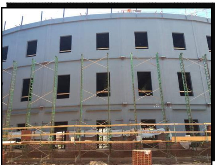
PICTURED ABOVE & RIGHT: WEATHER BARRIER, SHEATHING, AND FRAMING ALONG THE NORTH AND EAST EXTERIOR WALLS
