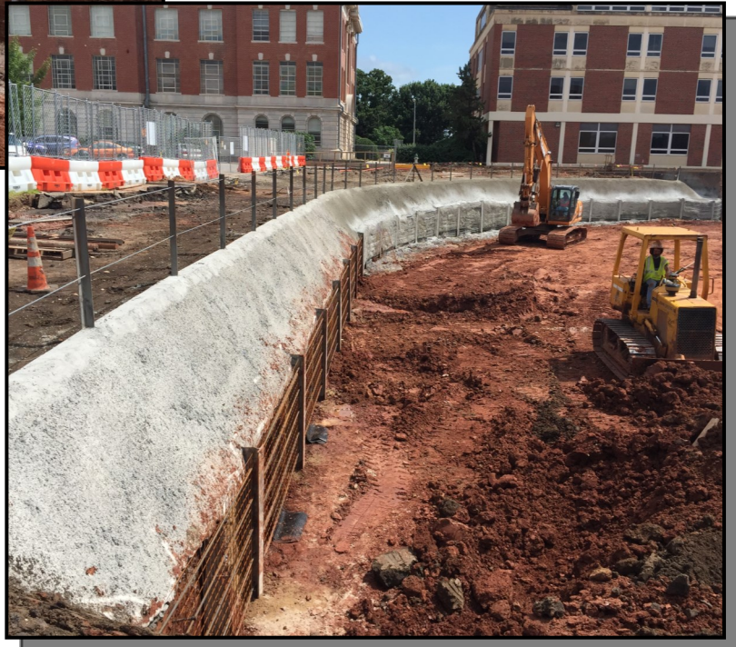
PICTURED: SHOTCRETE RETENTION SYSTEM IN- STALLATION
