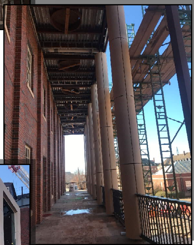
PICTURED BELOW: EAST CURTAINWALL GFRC INSTALL
