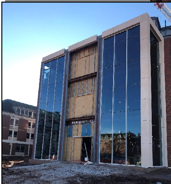
PICTURED BELOW: EAST CURTAINWALL GFRC INSTALL
