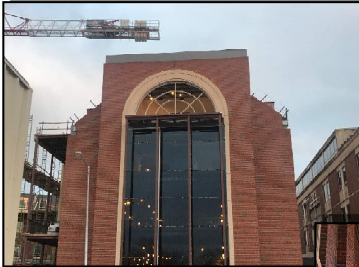
PICTURED ABOVE: NORTH EXTERIOR END CAP GFRC
