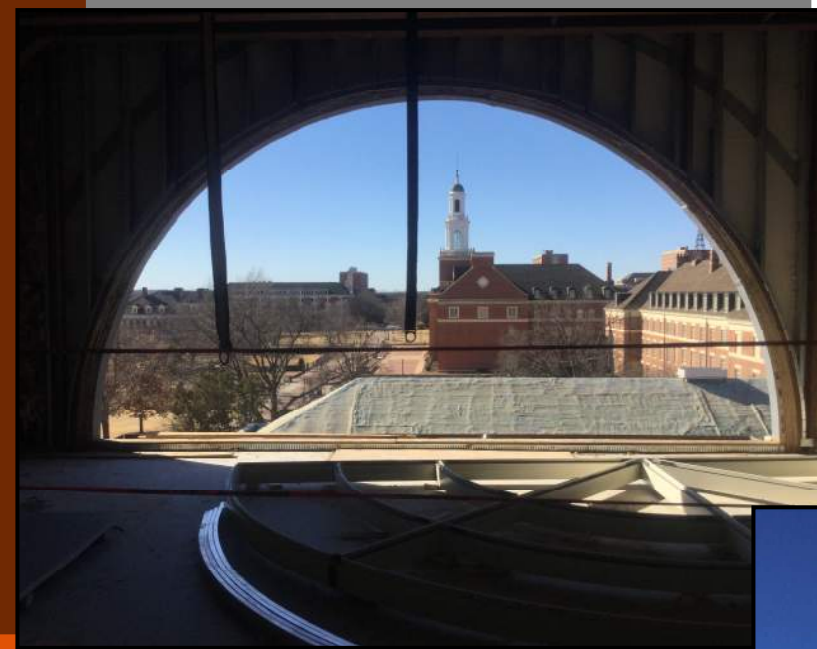
PICTURED ABOVE: CRESCENT/ROSE NORTH WINDOW INSTALL
