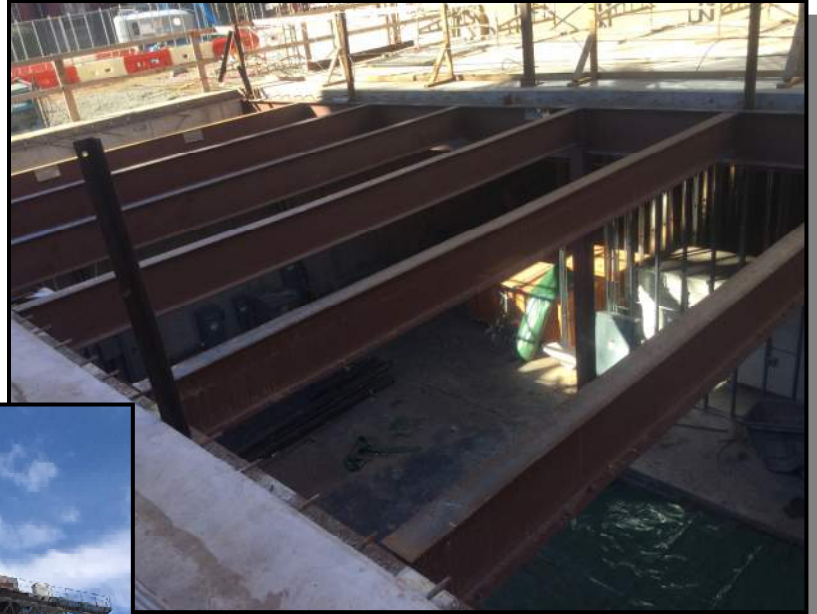
PICTURED ABOVE: LOGGIA PAD STEEL INSTALL
