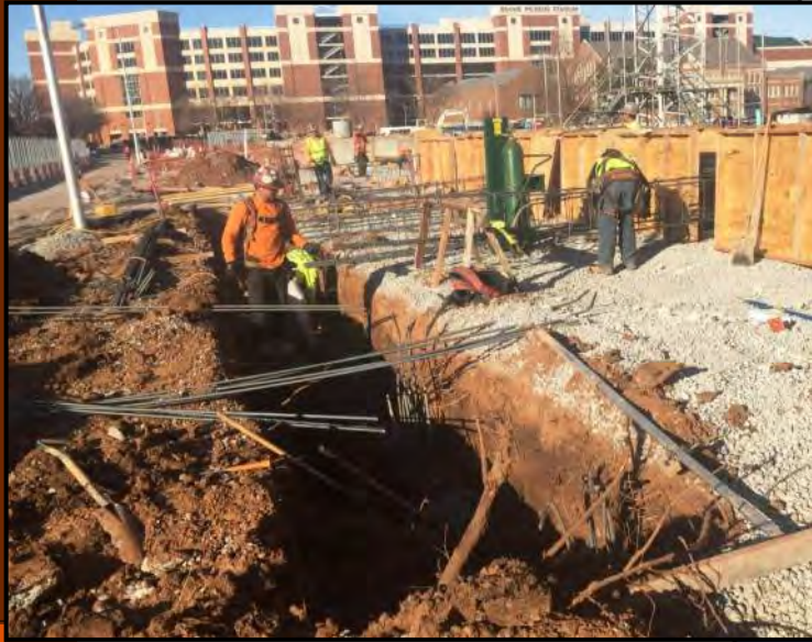
PICTURED BELOW: GRADE BEAM FORMS BEING INSTALLED
