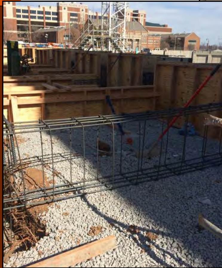
PICTURED BELOW: GRADE BEAM FORMS BEING INSTALLED
