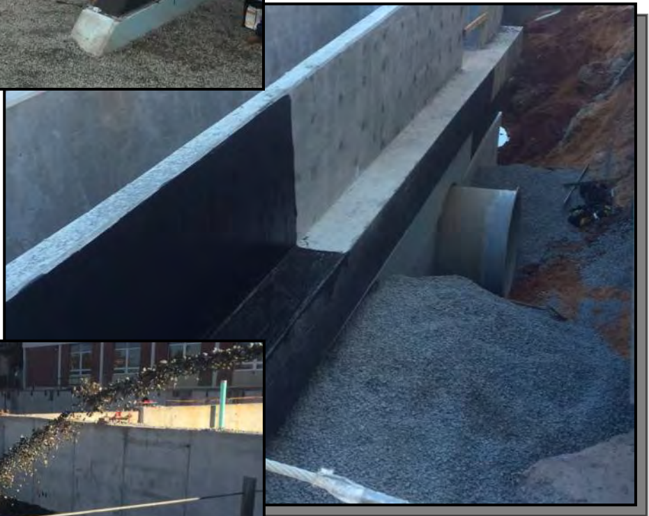
PICTURED LEFT: USING A ROCK SLINGER ALONG HESTER TO BACKFILL
