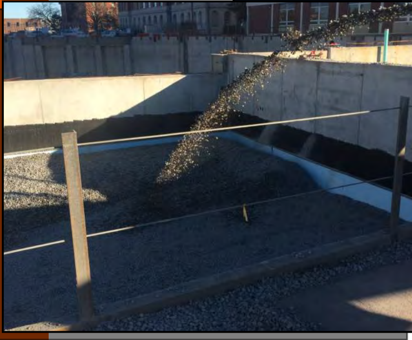
PICTURED LEFT: USING A ROCK SLINGER ALONG HESTER TO BACKFILL
