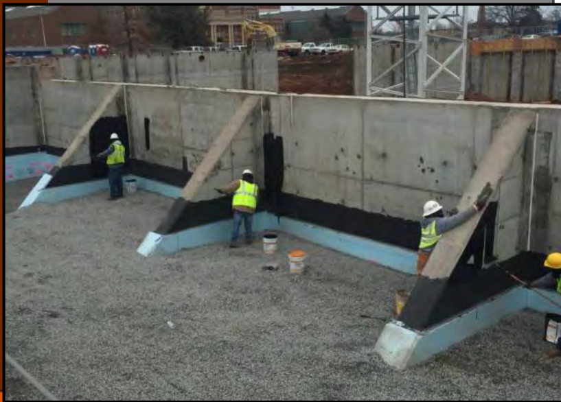
PICTURED LEFT & BELOW: INSTALLING WATERPROOFING
