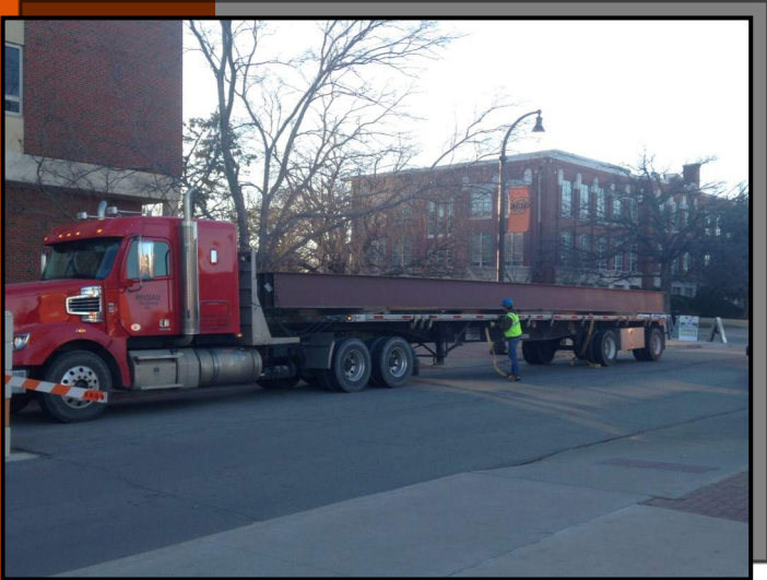
PICTURED ABOVE: STEEL BEING DELIVERED
