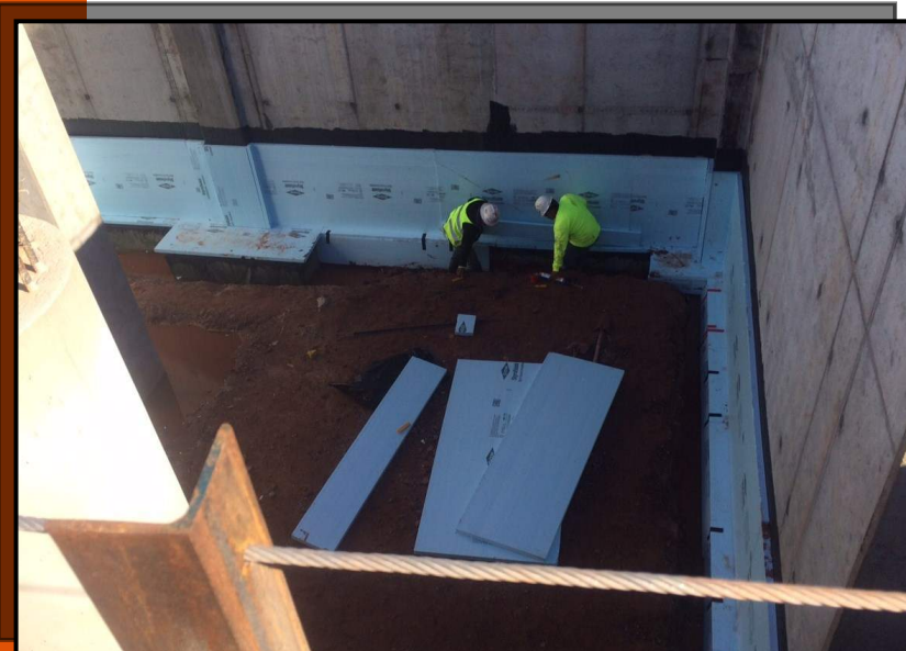
PICTURED LEFT: INSTALLING WATERPROOF- ING INSULATION BOARD
