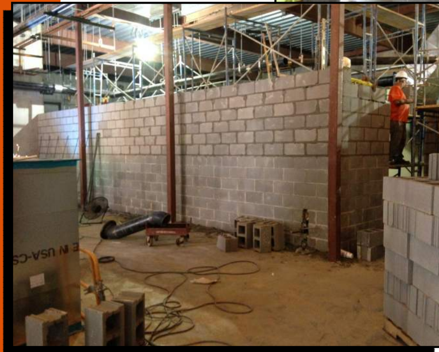
PICTURED ABOVE: SOUTH DECKING DORMER ROUGH IN PICTURED RIGHT AND BELOW: NORTH BASEMENT CMU MECHANICAL ROOM
