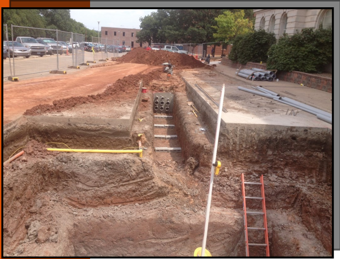
PICTURED: INSTALLATION OF ELECTRICAL VAULT NORTH OF MORRILL HALL
