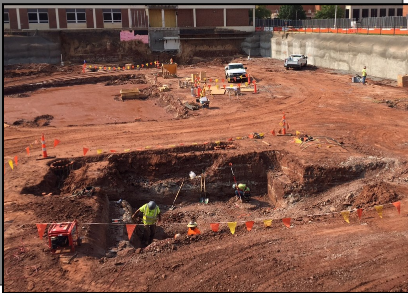
PICTURED ABOVE: EXCAVATION OF ELEVATOR PIT
