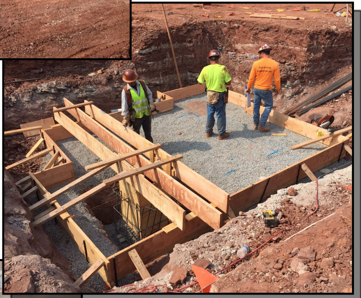
PICTURED ABOVE: EXCAVATION OF ELEVATOR PIT
