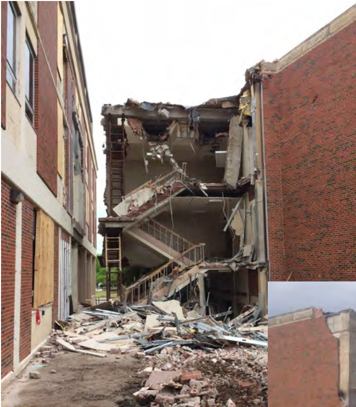
Pictured Left: Separating the Stacks from the Building to Remain
