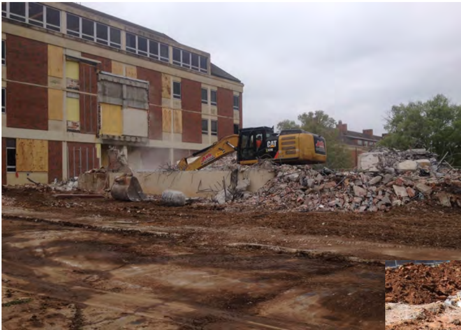
Pictured Left: Demo of Stack Basement Walls
