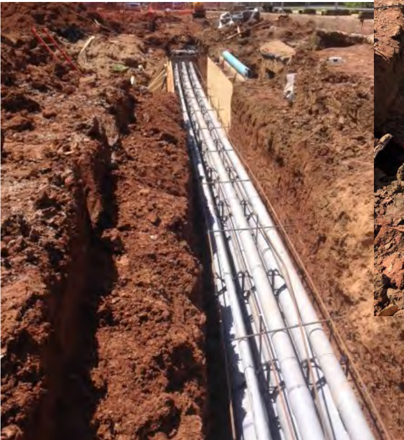
Pictured Left: Morrill Street Utilities Electrical Duct Bank Installation
