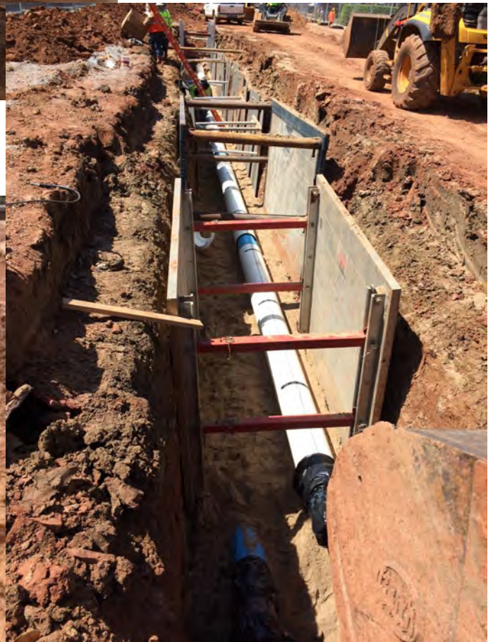
Pictured Below: Morrill Street Utilities Chilled Water Installation
